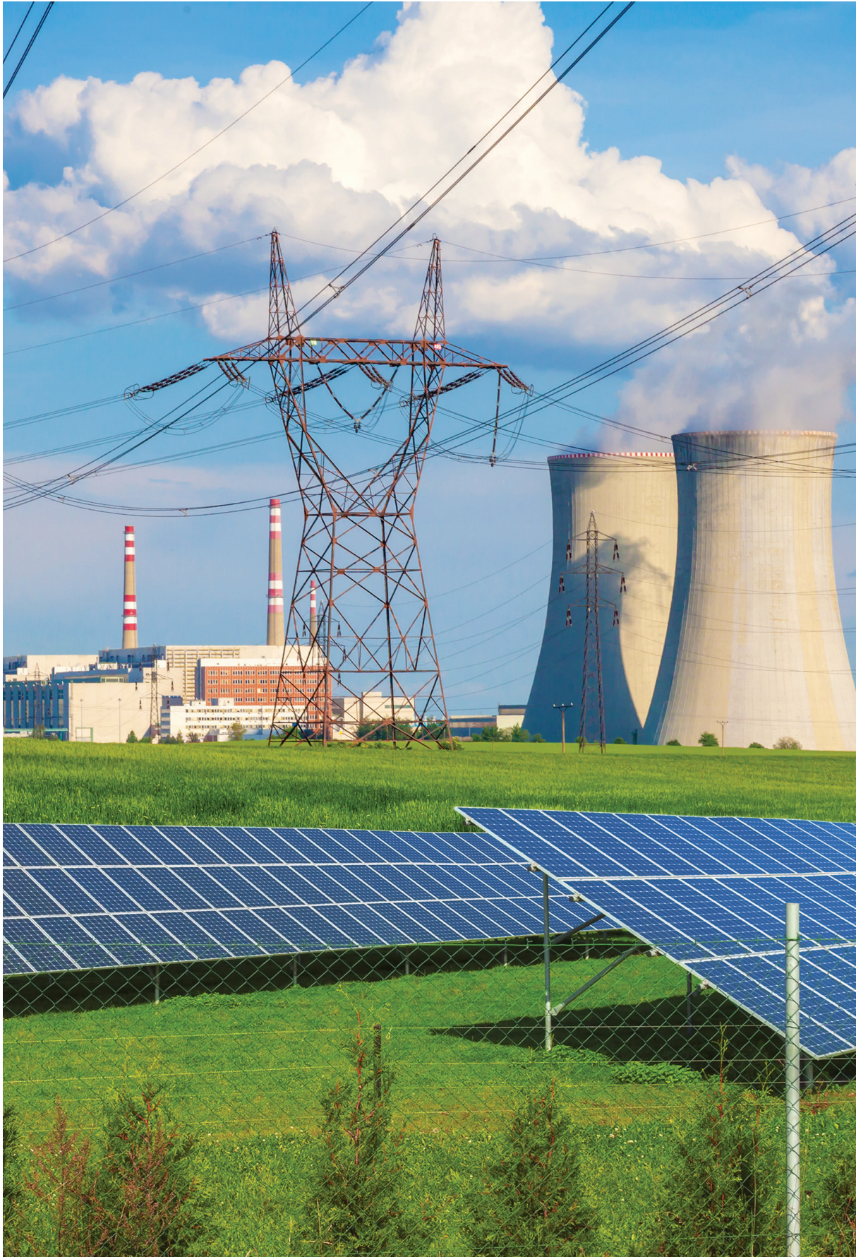
Dukovany solar and nuclear power facility in Czech Republic Martin Lisner
